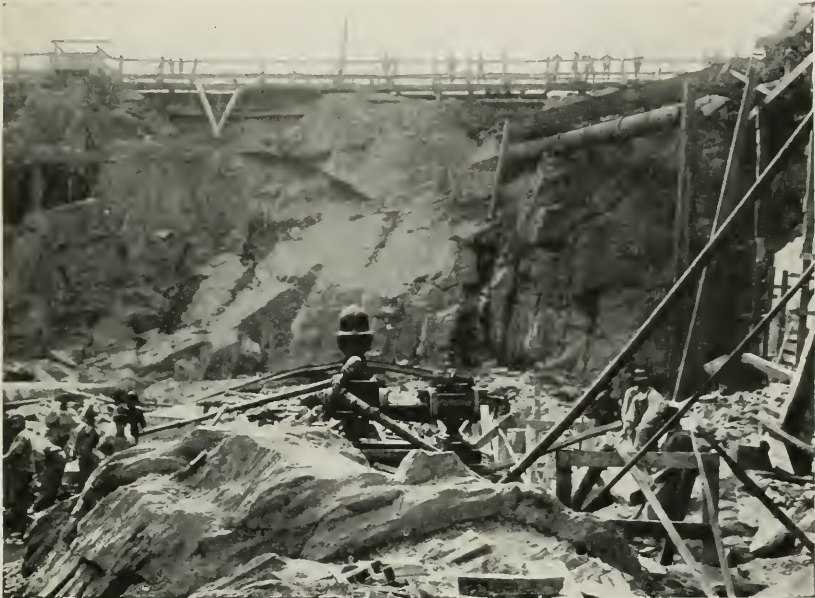
Looking east at Seventh Avenue. Approach to new Pennsylvania Terminal, with Cameron Pump removing 400 gallons drainage water per minute from the diggings to the sewer 65 feet above.
